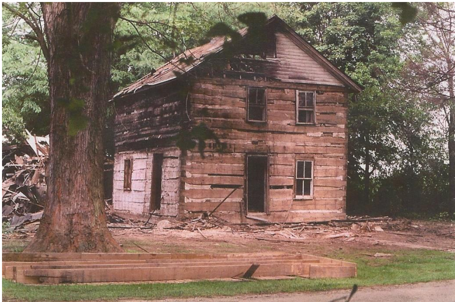
Morgan Leonard House being dismantled
