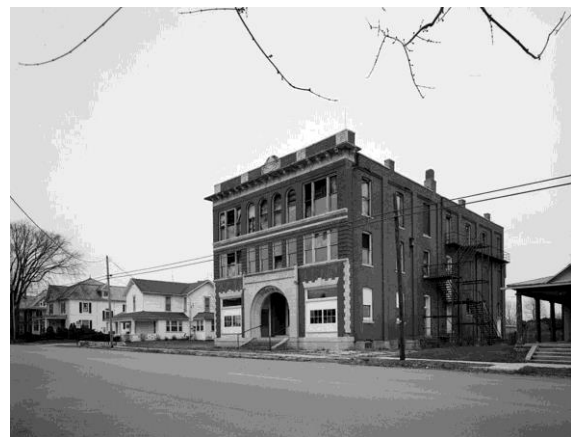
Last picture before demolition
