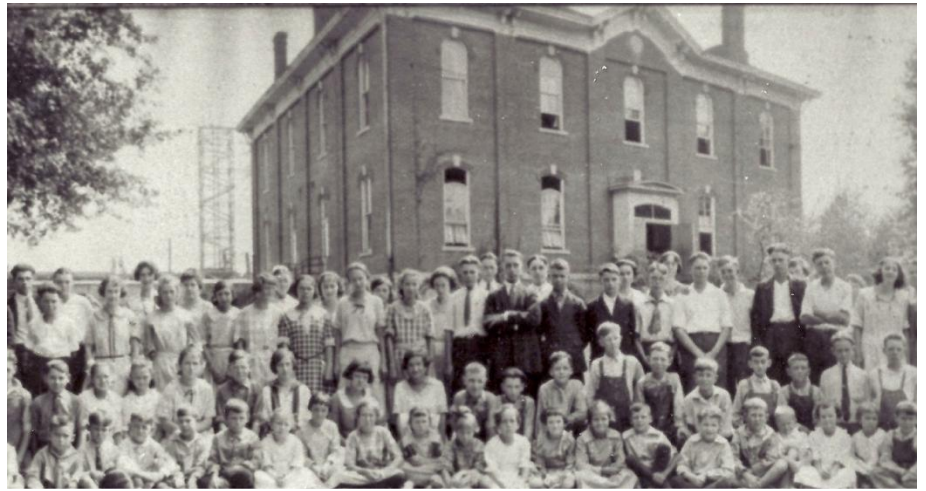
Scaffolding for the new building can be seen behind the 1875 building.
