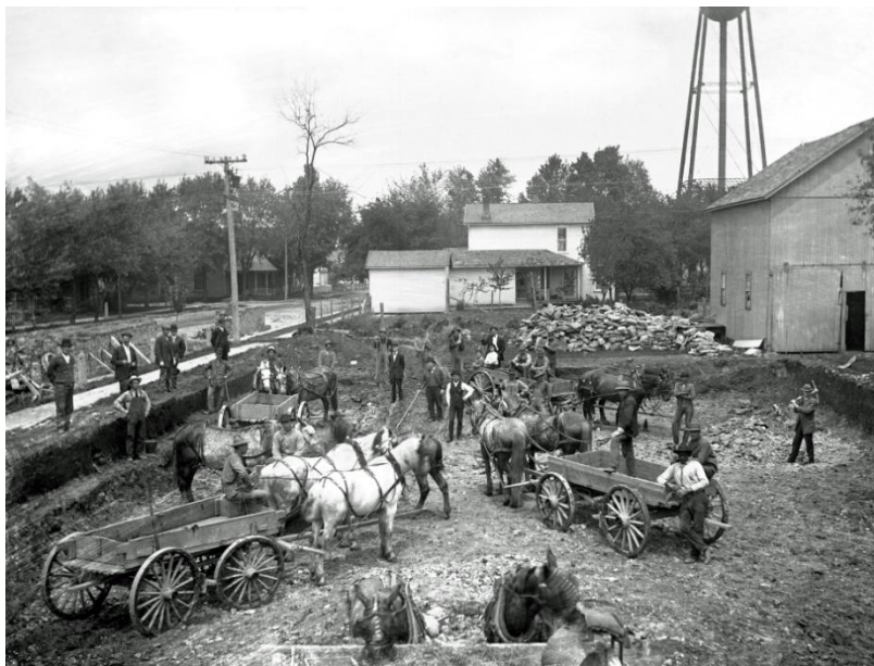
Digging the basement of the 1910 church
