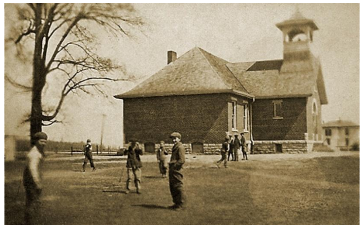
Pattytown 2 room school built in 1904
